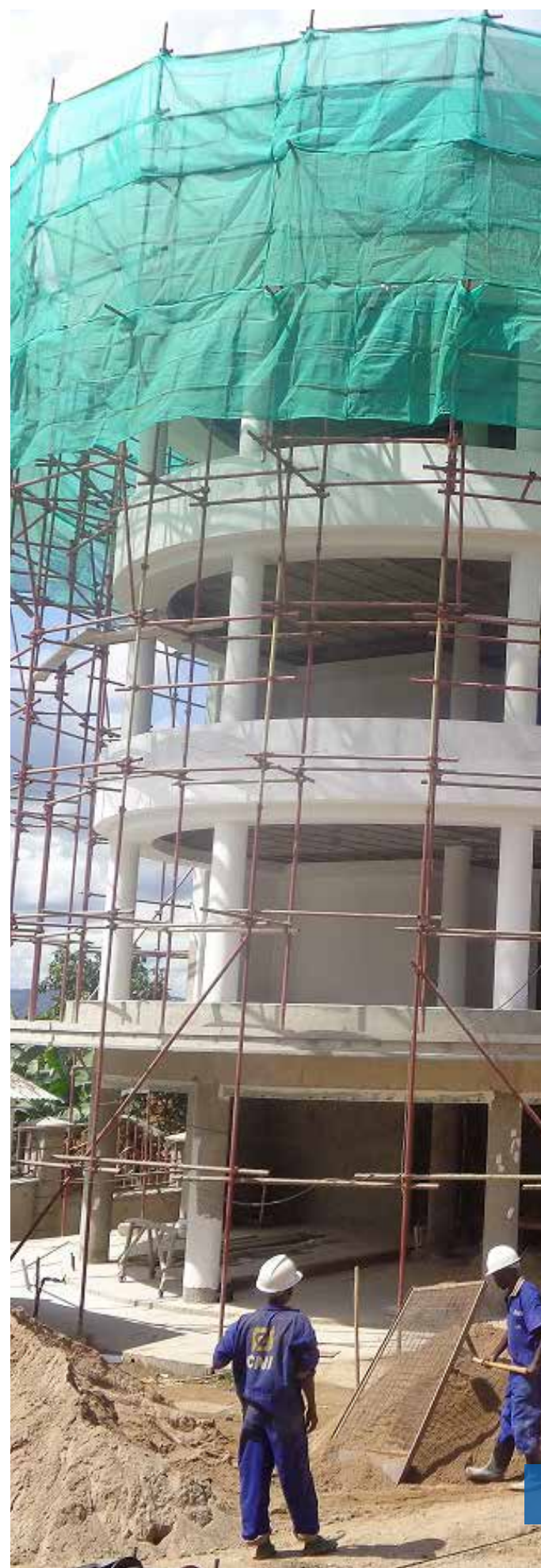
NSSF Mbarara City House Building under construction
